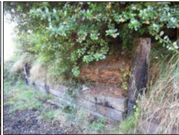
Figure 4. Deteriorating timber pile wall along the lower part of the beach access roadway. Note creosote pile.
